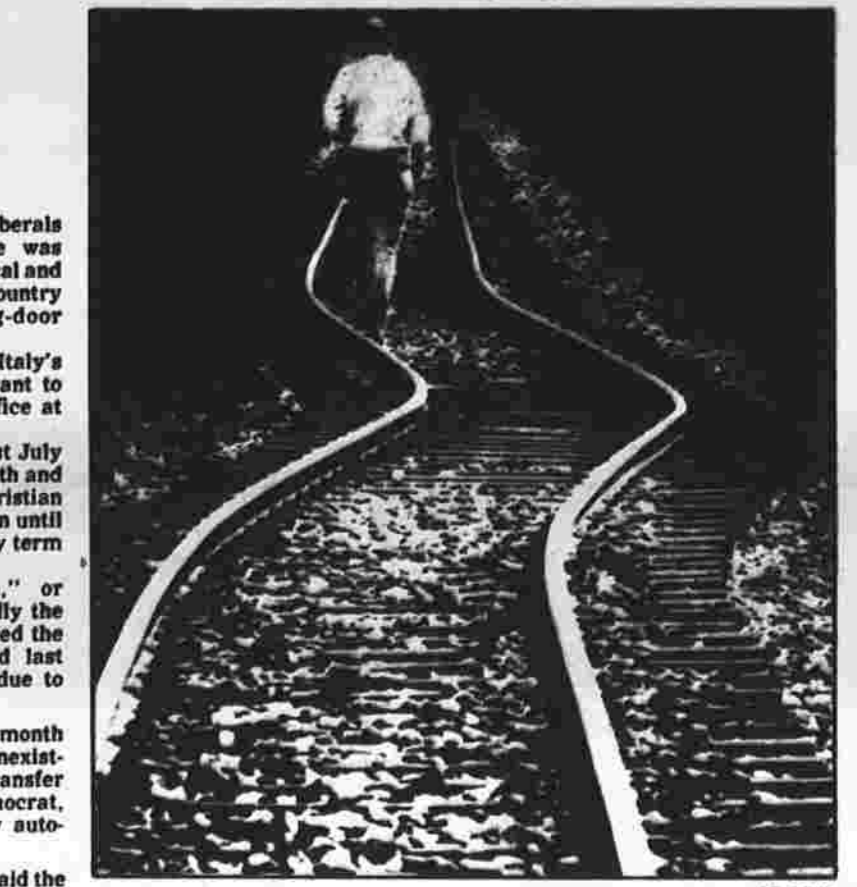
Quake damage A man walks along railway lines on the North Island of New Zealand that were buckled by an earthquake Monday. The quake, which centered about six miles offshore, registered 6.5 on the Richter scale.
